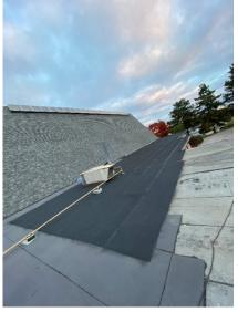
Due to water damage caused by poor drainage on the flat roof it was decided to invest some money in this area and remedy the flaws for good. Most of problems were caused by the water staying on the roof in large puddles. Contractors were hired to build a frame that would have a gradual slope that enabled the
